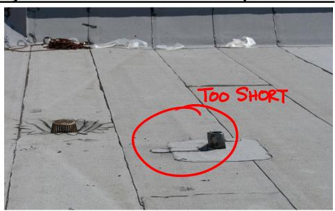
Pipe was cut short because the roof insulation was not taken into account.
