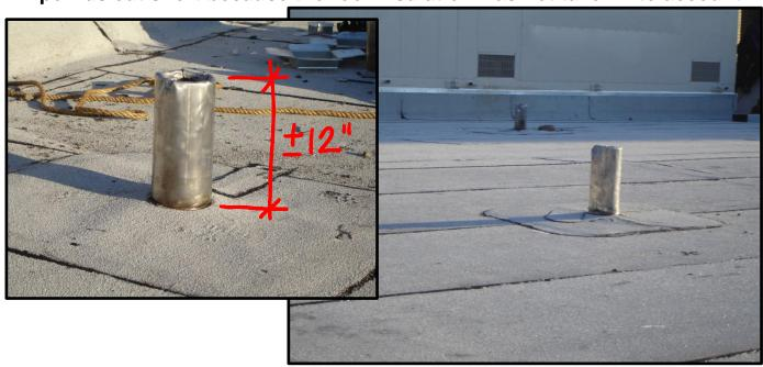
The Pipe should be about 12" (IL Plumbing Code 089.1430a) or more above the finished elevation of the roof.
